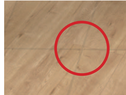
Traditional vinyl flooring: Irregularities caused by old sub-floors may show on the surface
